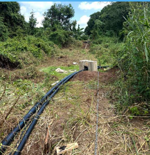
Installation of piping system to the farms to improve access to water | Photo UNDP CRRF
