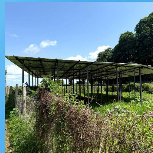
Solarization of the pumping system in an irrigation scheme in Kenya | Photo UNDP CRRF
