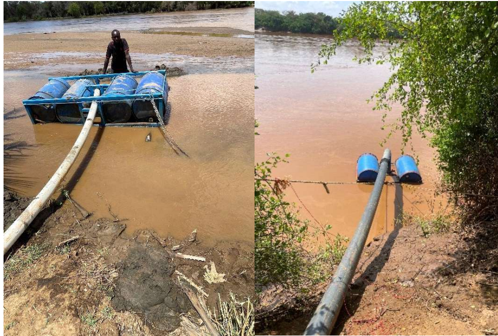
Pontoon System at Ngao irrigation scheme Photo: UNDP CRRF
