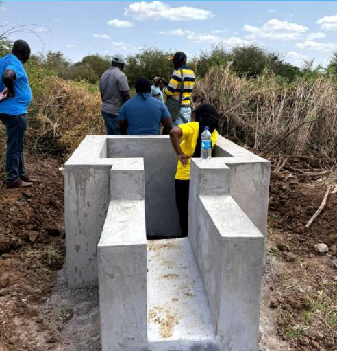
Construction of the distribution channel to the farms | Photo UNDP CRRF
